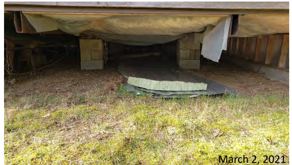
Photo 14 – Existing mobile home supported on concrete cinder blocks.
