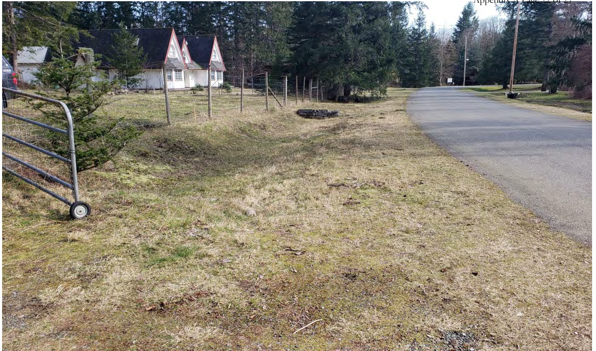
Photo 17 - Swale along Riverbend Road.
