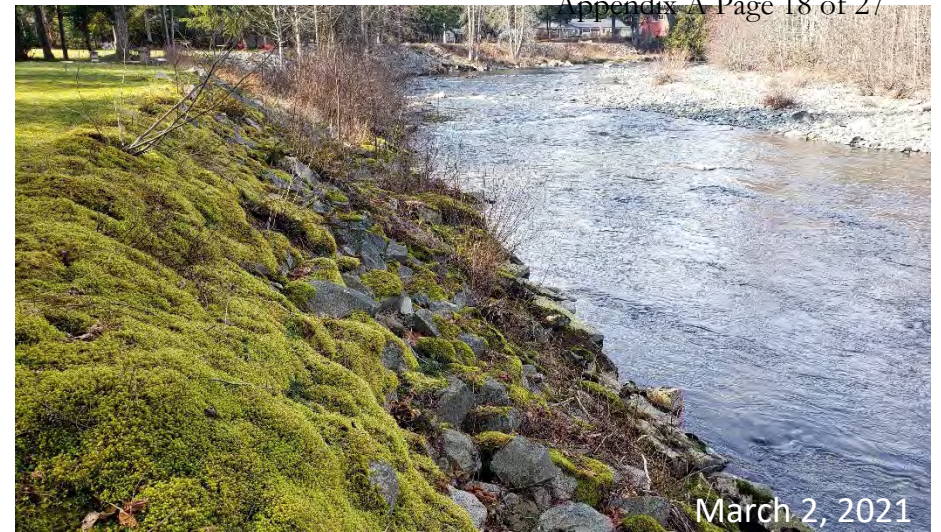
Photo 8 – Looking upstream at rock armouring on bank.
