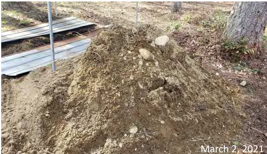
Photo 13 – Sandy material stockpiled from test pit containing some cobbles.
