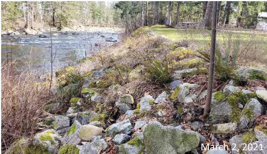
Photo 3 – Oyster Riverbank rock armouring in front of subject property looking downstream.
